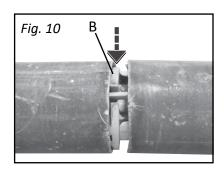
**6**. Push down on stop (B) until it rests underneath inside of pipe. (Fig. 10)
