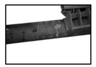
5. Continue to bend pipe to desired angle, placing the bending shoe on marks made in
